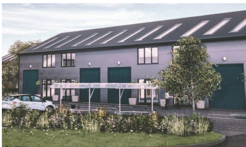
Figure 45 – Apollo Technology Park, Wellingborough (Source: Apollo Park)
